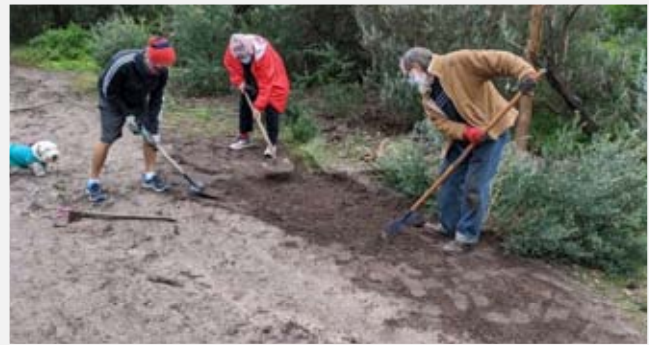
Our emergency volunteers filling in deep holes made by trail bikers to create an 'interesting' track .
